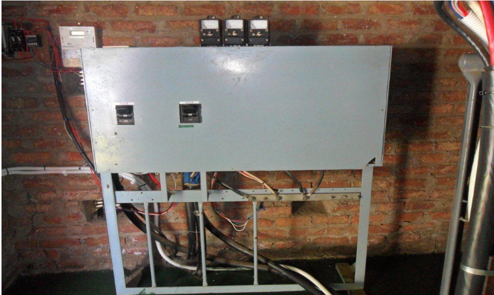
LV MCBs board made of chipboard and other MCB against the wall.
