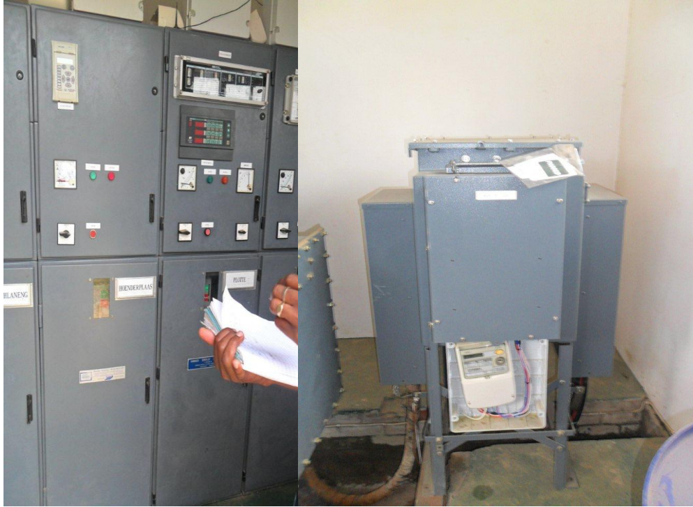
Indoor oil breaker in good condition with and compact T3 switch
