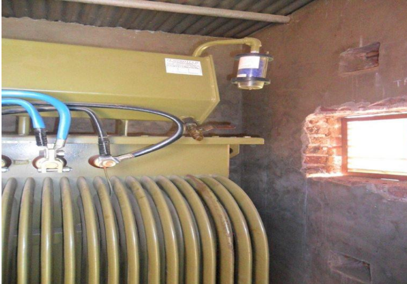
Transformer and silica gel in good condition
