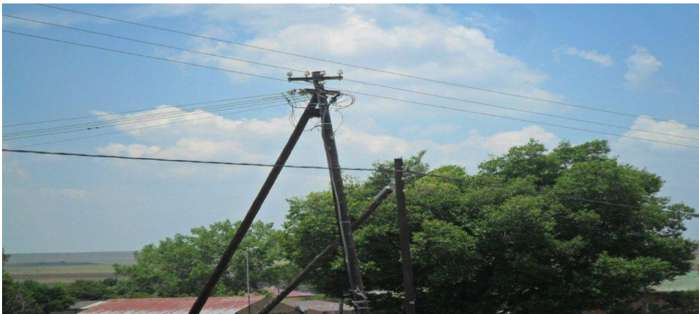
LV line upgraded with new poles & bundle conductor correct clearances between MV and LV line
