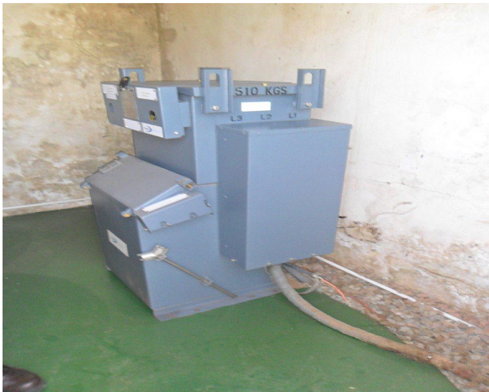
New T3 switch in good condition
