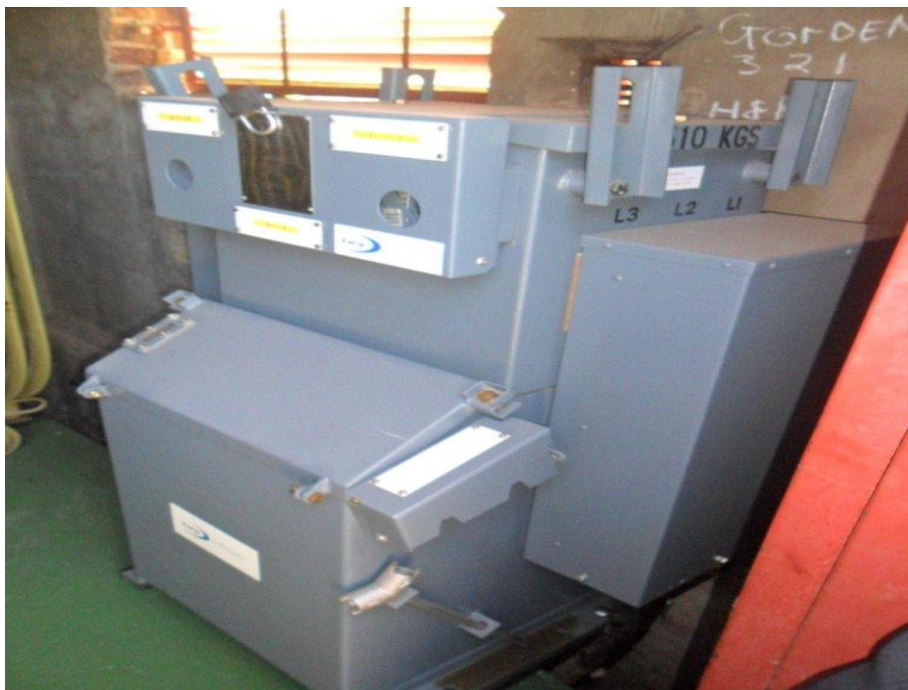
New T3 switch in good condition
