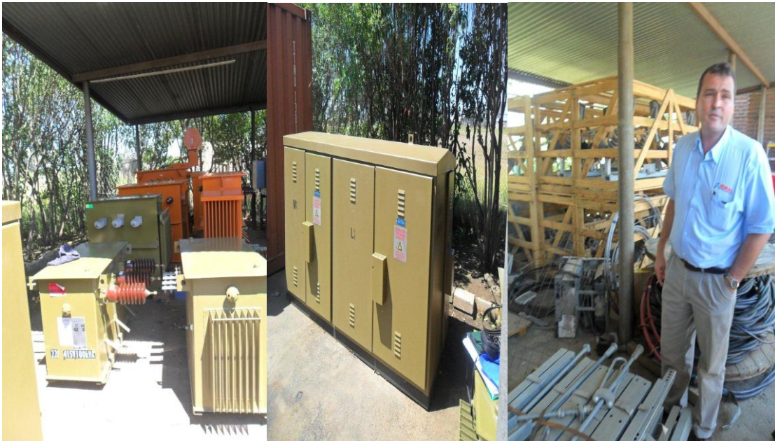
Spares in stores mini sub, transformers, bundle OH conductors and other ancillaries
