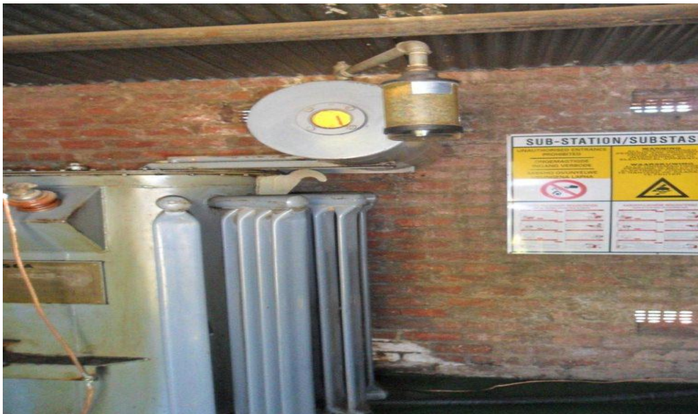
Transformer and silica gel in good condition
