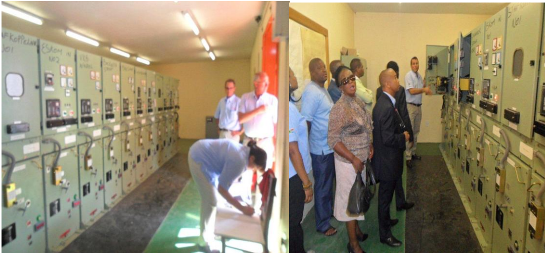
New sf6 Indoor breakers in good condition
