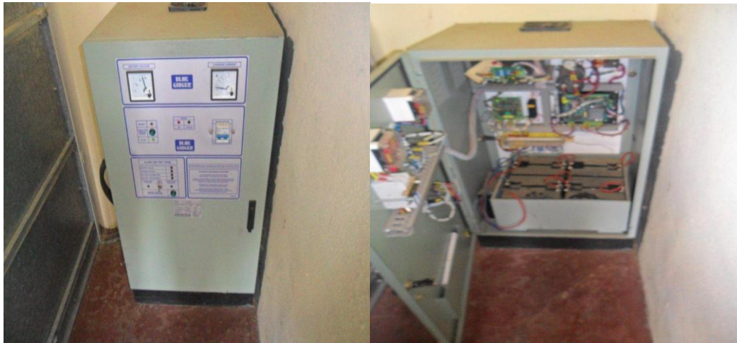
Battery charger with dry cells inside all in good condition
