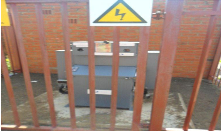
New T3 switch on cement plinth inside barricade with warning sign
