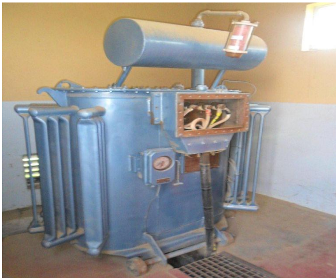
Transformer and silica gel in good condition
