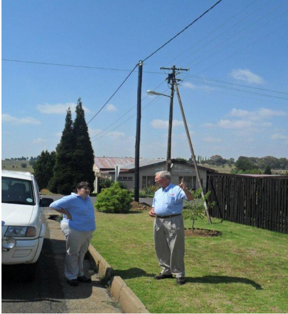
New LV bundle line installed
