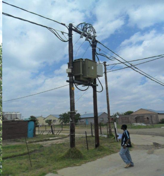
Pole transformer in Tweeling in good condition
