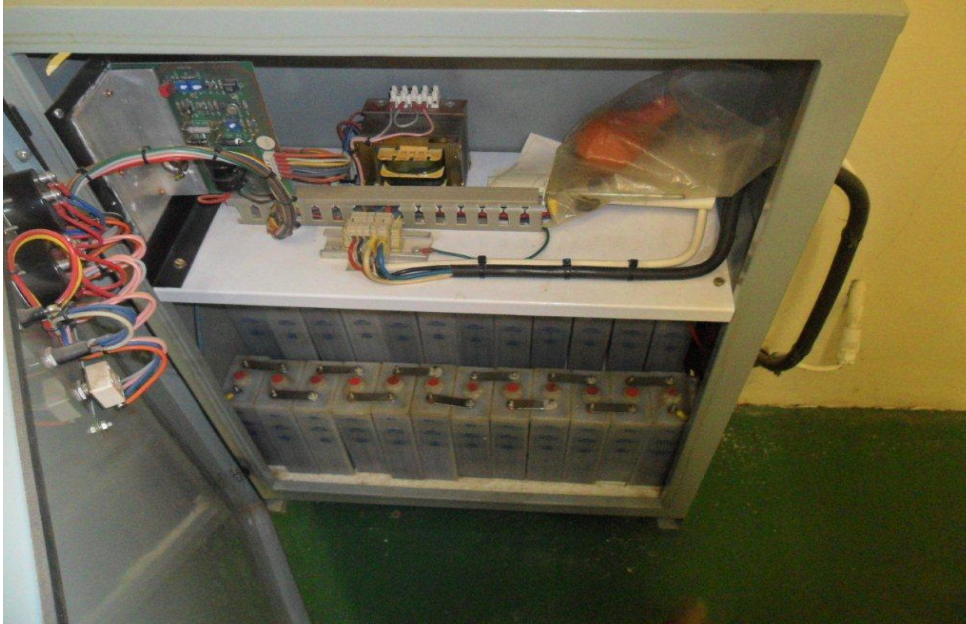
Battery charger in good condition with low battery levels
