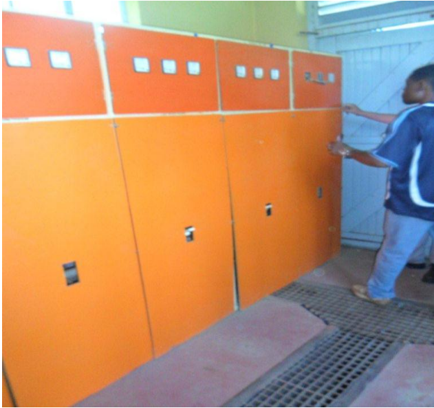
LV MCBs board made of chipboard and not properly labelled.
