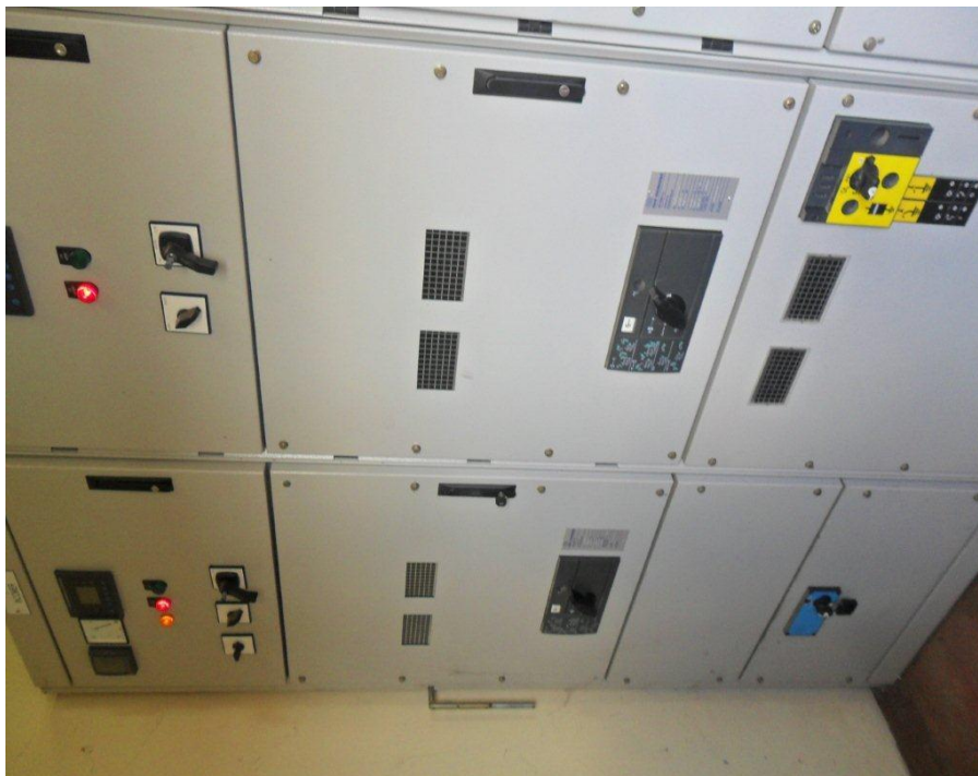
Indoor breaker in good condition with
