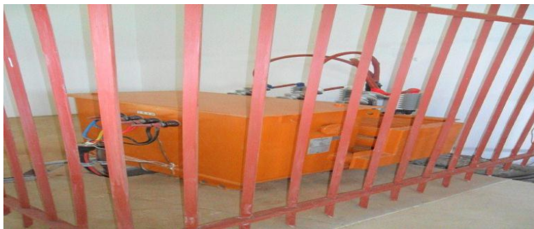
New transformer and silica gel in good condition with surge arrestors
