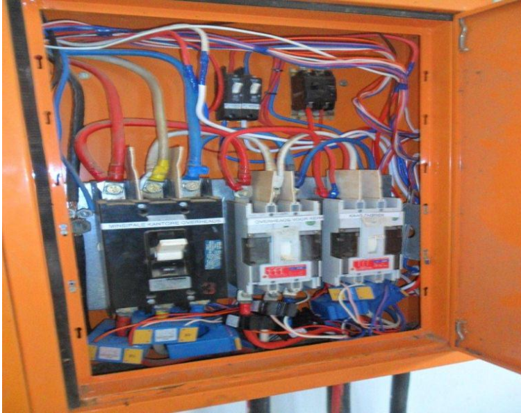
Proper LV MCBs cabinet in good condition and properly labelled.
