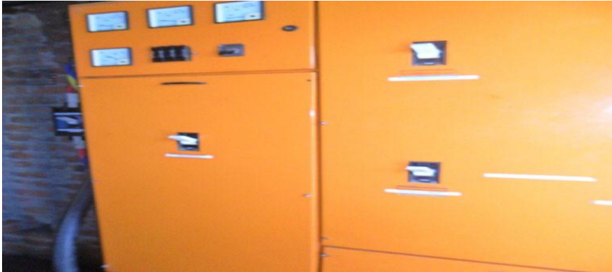
MCB mounted against the wall next to proper panel with designated LV MCB
