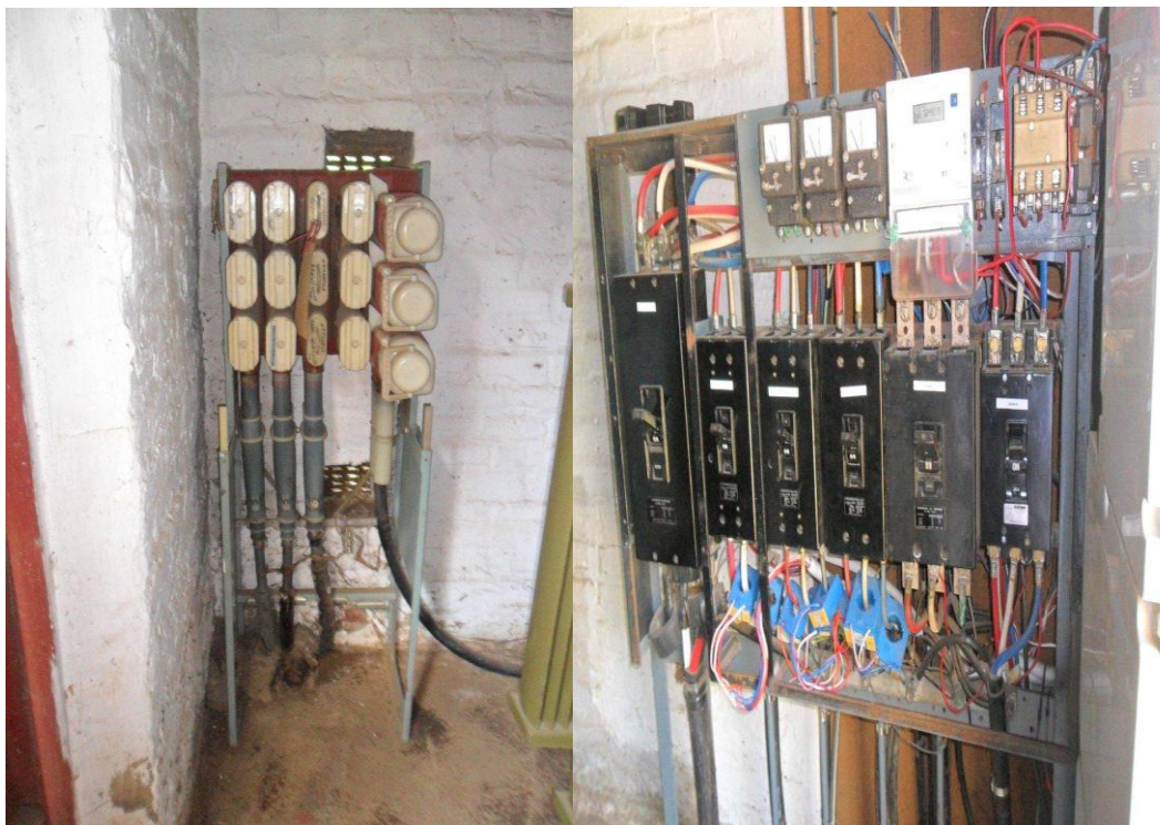
Old magenfix switch LV board with MCB mounted against wall on a frame
