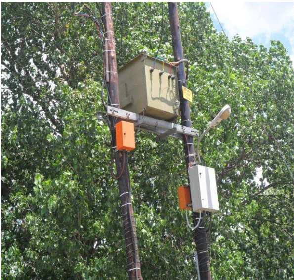
Pole transformers at Villiers in good condition with coms
