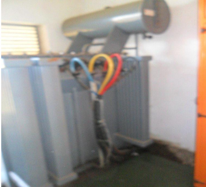
Transformer and silica gel in good condition
